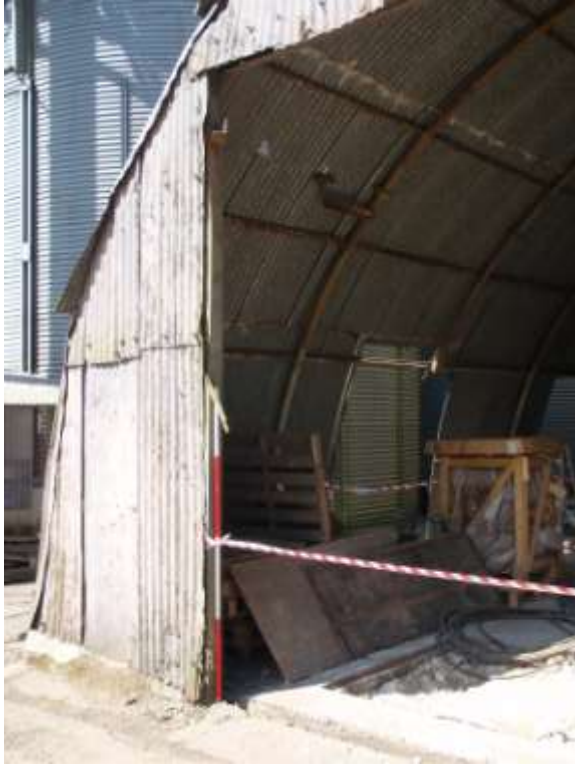
Plate 3. Front view(looking NNW)
