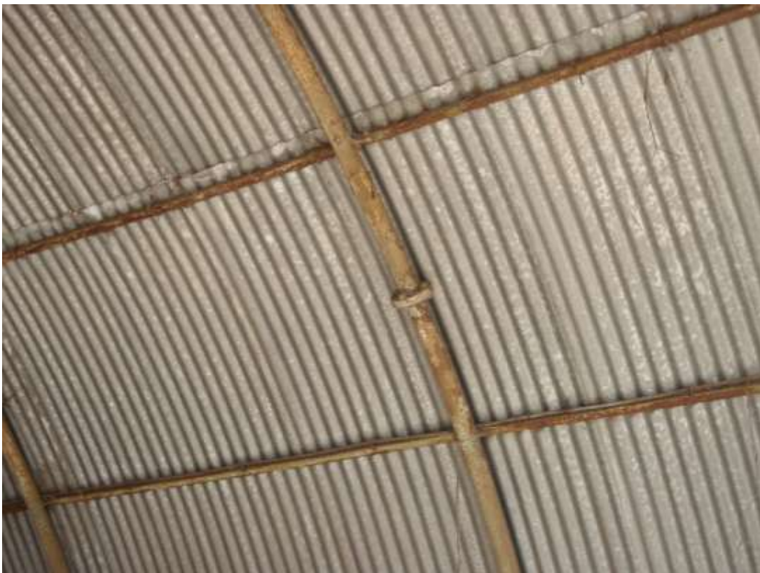
Plate 6. View of struts
